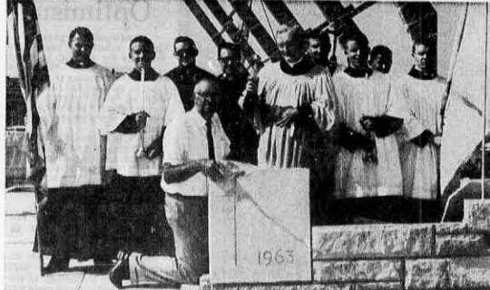
AT COLUMBUS CEREMONY —The Very Rev. Omer Eisenman, V.F., dean of the North Vernon Deanery (center in surplice) blesses the cornerstone for the new St. Columbus's Church, Columbus, Ind. Al Graffa is setting the stone in place. The two priests behind Mr. Graffa are Father Patrick Gleason, right, pastor of St. Bartholomew's Church and organizer of the new parish, and Father Donald Schweizer, assistant pastor at St. Bartholomew's. The cornerstone rite was held last Sunday.
