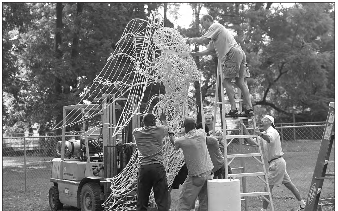
Friends help Patrick Mack secure the steel angel sculpture on a forklift before lifting it onto a pedestal in his backyard. The sculpture faces the Monon Rail-Trail, a public-access exercise route, at 5000 north in Indianapolis.
