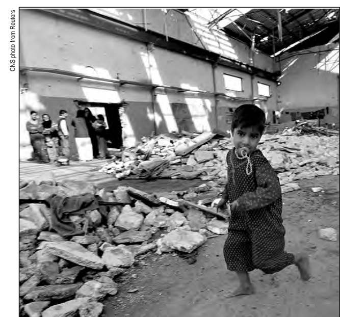
An Iraqi child plays amid the rubble of a former rocket factory that was hit by bombs in Baghdad during the U.S.-led war. In December, at least 10 homeless families were occupying the damaged building. The invasion came in mid-March despite the U.S. failure to win U.N. support and over the objections of many religious leaders, including Pope John Paul II.
