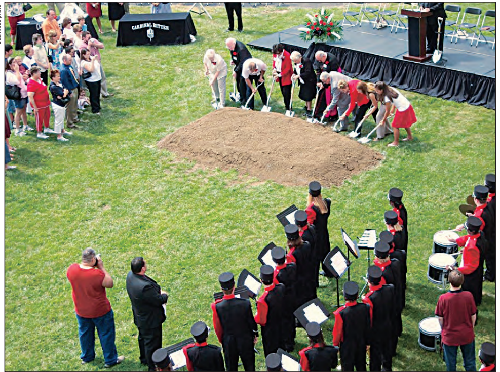
Cardinal Ritter Jr./Sr. High School students, faculty, administrators and supporters break ground on June 21 to inaugurate the construction of a new Fine Arts wing and chapel at the Indianapolis West Deanery interparochial high school. The school is using a $1 million allocation of a Lilly Endowment grant to the Archdiocese of Indianapolis to make capital improvements.
